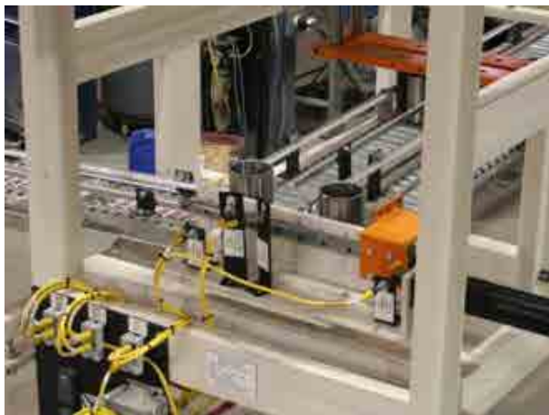
Piston Liner Gravity Feed Conveyor With Meter and Turn Lanes
