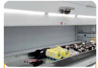
External Bay Lighting
