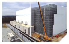
In clad-rack buildings, the racking forms part of the structure of the building.
