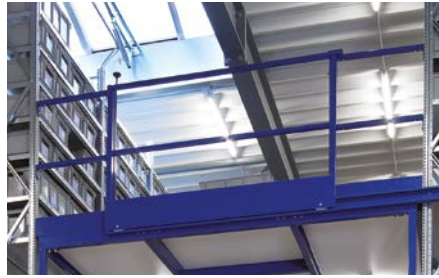
Transfer station with sliding gate
