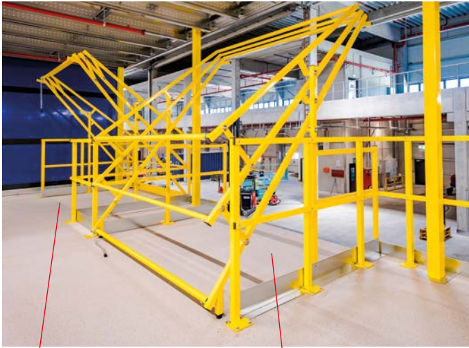
Pallet gate open
