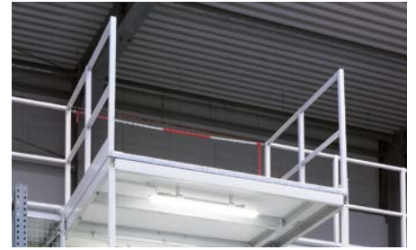
Transfer station with chain
