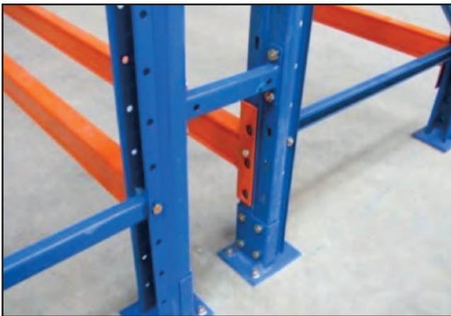
Example of roll formed row spacer
