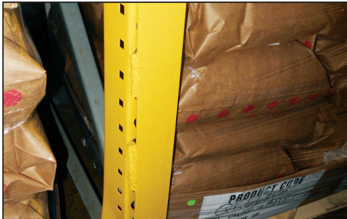
Non-engineered repairs
