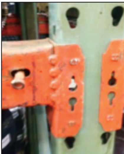
Missing / damaged safety-locks
