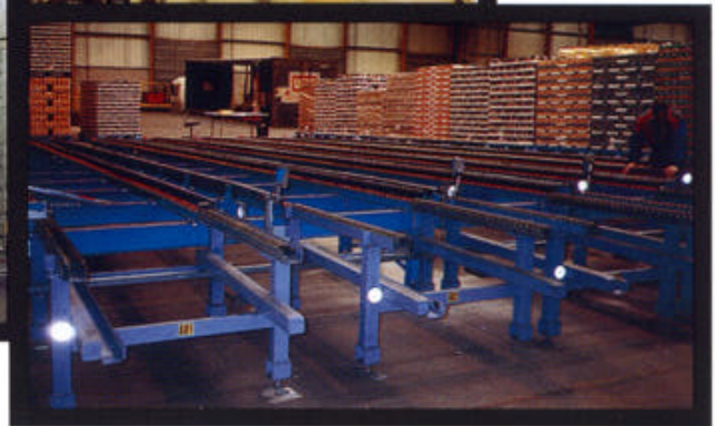
Truck Staging England
