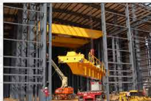
75-Ton Double Girder Installation
