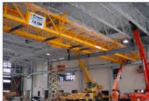
Truss Crane Install using 4 Mobile Cranes in a Critical Lift
