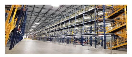
Gates are custom designed to the rack and mounted on the inside upright member. Systems can be custom designed for small, standard and very large bays
