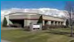
INTERSTATE GRATINGS, UT ▲
