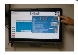
with energy efficiency year-round. Tudor and his team can manage the fans from the all-in-one, high definition touch screen computer located in a locked storage area accessible only by authorized maintenance personnel. The controls even include custom graphic displays of the facility and fan locations to easily pinpoint a fan's exact location if adjustments need to be made.
