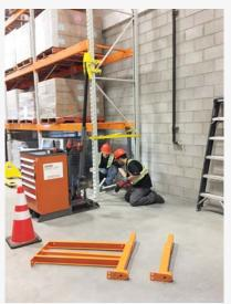
Thanks to the EASY LIFT, the installation of a rack repair kit requires minimun unloading and is non disruptive to your operations.
