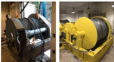
25 Ton intake gate winch replacement for an energy client's dam
