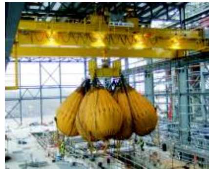
Overhead Bridge Cranes
