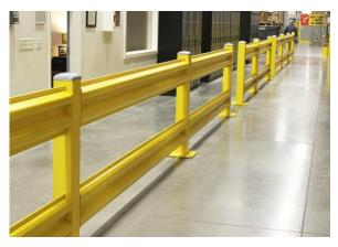
critical functions (i.e. receiving and dispatching products). Additionally, micro-fulfillment centers that choose to install a mezzanine will also need to invest in products like guard rail and safety gates (two traditional material handling staples) to ensure that the platform's elevated ledge is protected.
