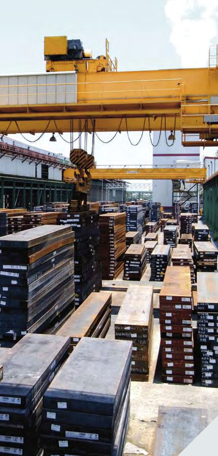
Below: Slab storage crane. Right: Coil handling crane.
