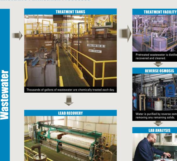
olids are removed, smelted and refined for lead recovery.
