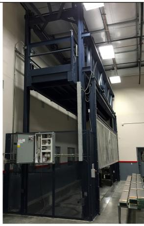
largest engineered and fabricated gates of its kind by PFlow Industries. On the second level, the load exits the lift 90° through an opening with a steel roll-up door; the same narrow opening the forklift had previously used.
