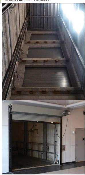
An F Series, four-post VRC runs the 73' distance from the ground floor to the sixth floor Service Department, with stops at each level in between. It has a useable lift carriage of 10' 0" W x 20' 0" L x 8' 0" H and an 8,000 lb. capacity. Primarily intended to move inoperable cars to the storage and service levels, it features powered steel roll-up doors at each level and plenty of capacity to lift Audi's largest luxury models.
