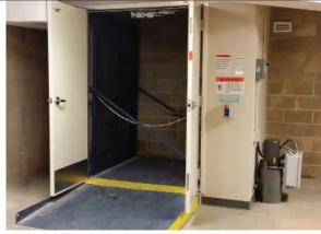
The E-ZPass D Series is a cantilevered frame design, with all structural elements attached to one basement wall, forming an L-shaped configuration with the lift carriage. The hydraulic pump and controller are stack-mounted adjacent to the lift, with a flexible hose connected to the two 2" ram direct-acting hydraulic cylinders that lower and raise the lift.
