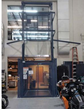
After a site visit and a requirements analysis, Florida Lifts recommended a PFlow 21 Series hydraulic VRC to better access Chester's FtL 14' mezzanine. The investigative process began in the Spring and the lift was installed by Florida Lifts later that Fall.
