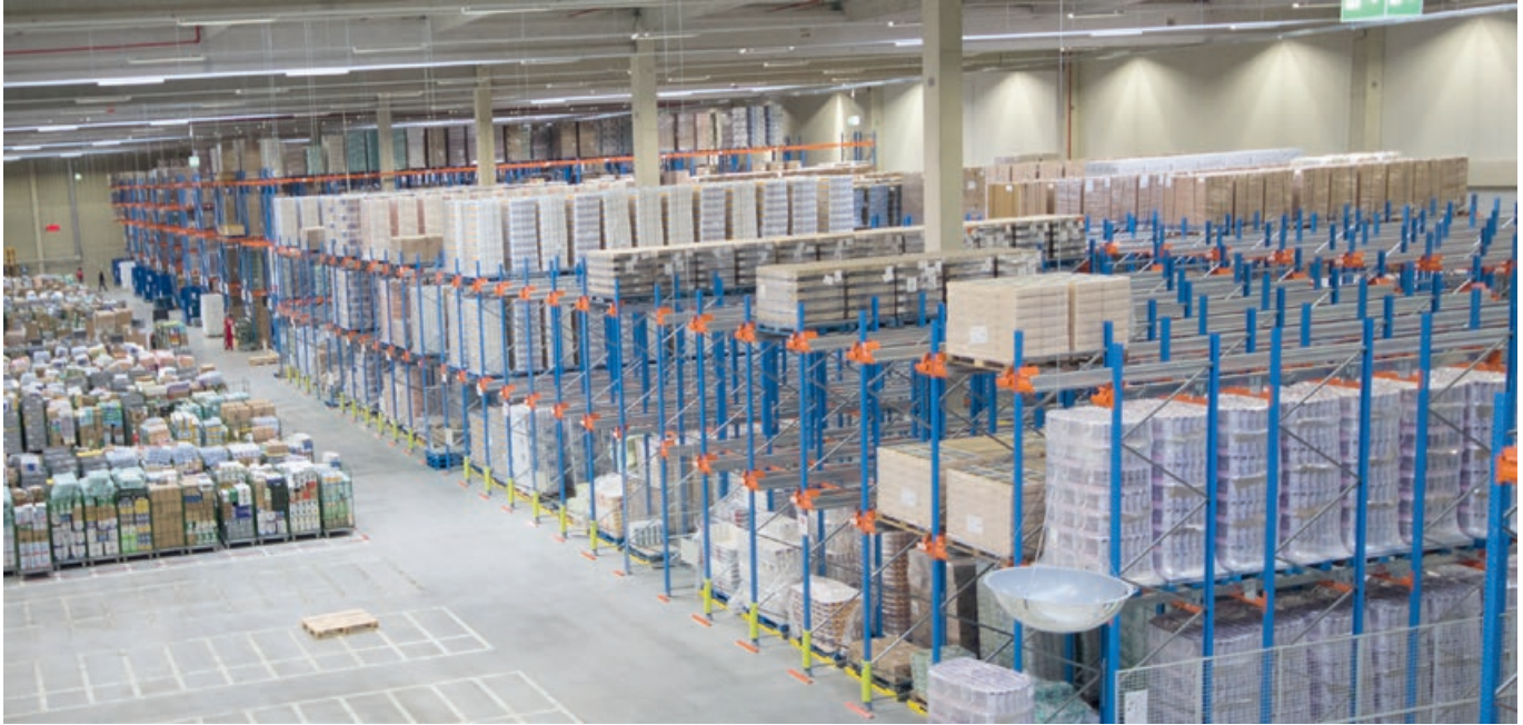
Shuttle warehouse with inclined roller track
