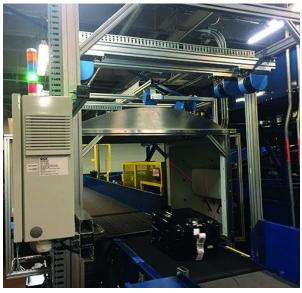
The RFID tracking system installed at Love Field provides a more efficient and cost-effective way to ease congestion in the CBRA area.
