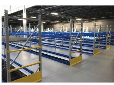
Ridg-U-Rak's highly efficient design uses ResinDek® with TriGard® flooring for a 3PL's rack supported platforms in two different warehouses.
