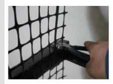
RackGuard pallet rack safety netting (more accurately described as Vertical Warehouse Containment Netting) is an engineered thermoplastic net (or grid) made from high performance polymers which produce high tensile strength and dimensionally stable meshes necessary to prevent warehoused goods from falling.
