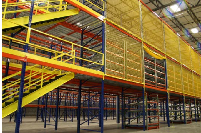
Pull rope raises/lowers safety gate
