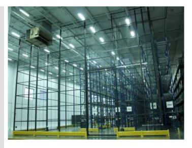
The DEA cage for this application was designed to be flush to the floor of the facility and to reach the roof deck of the building; some 40 feet high.
