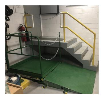
Payne and Atlantic Lift Systems also cut out a portion of the railing on the stairway landing and retrofitted it with PVC pipe so that equipment and supplies could easily pass through to the lift.
