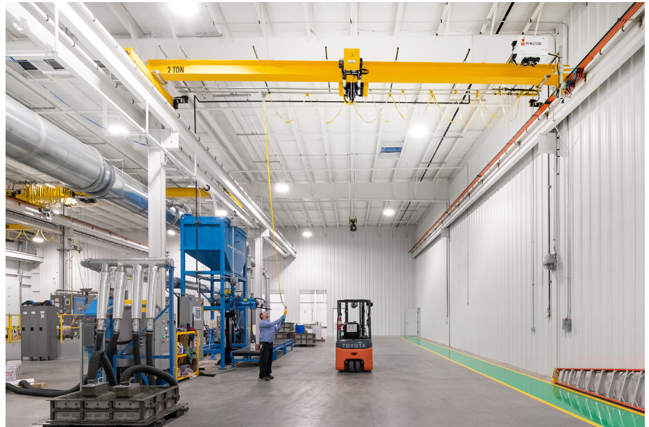
Single girder crane at Kimura's new rapid prototyping facility
