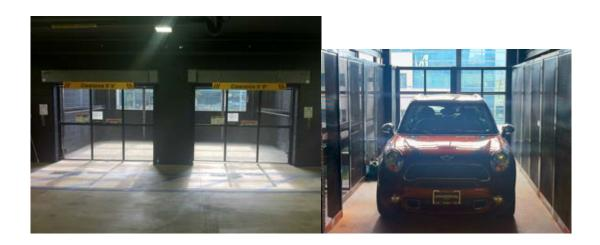
Two side by side 4 Post Mechanical Freight Lifts create a more efficient operation for a busy Mini Cooper dealership.
